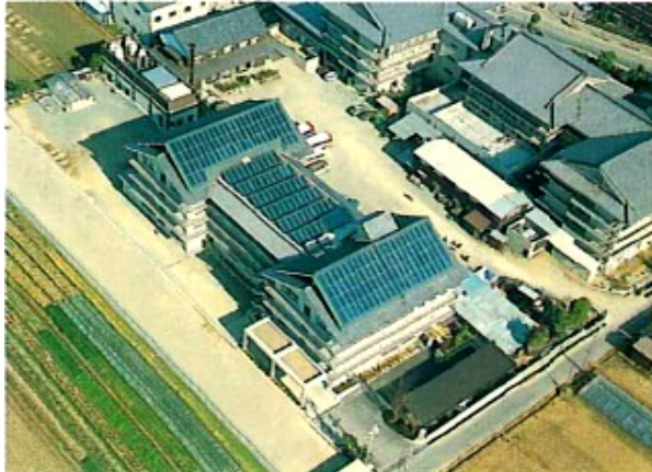
Solar Cooling 70 kW 1980
