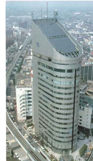
Solar Cooling 105 kW 1985
