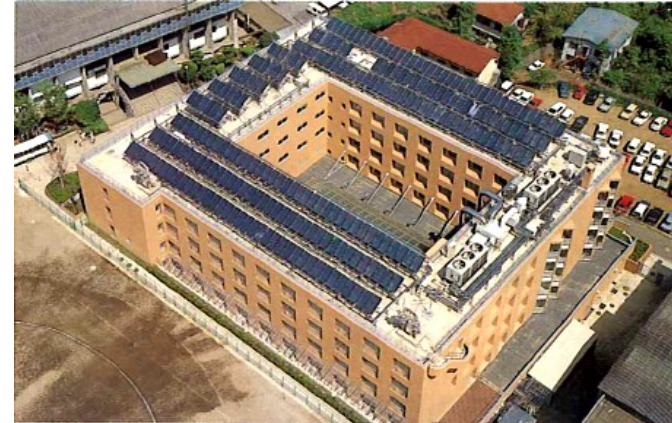
Solar Cooling 70 kW 1982
